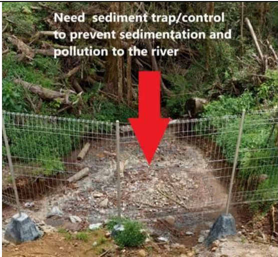
Drainage channel to river
