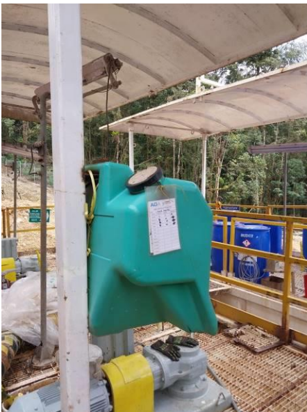
Emergency eyewash lack of Signage to indicate the position
