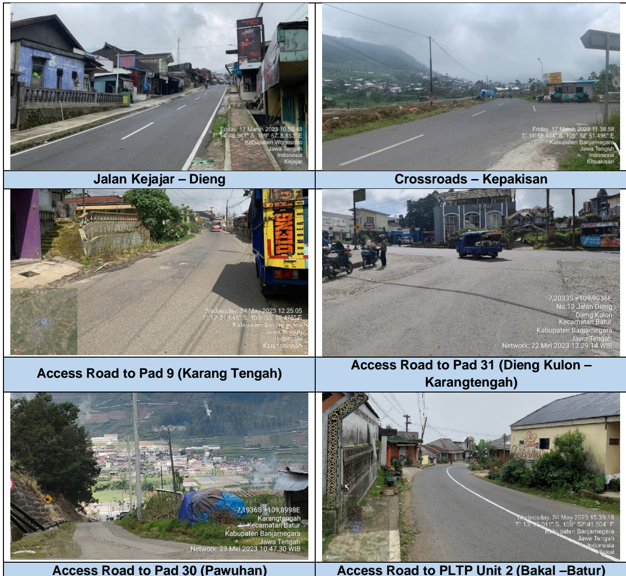
Figure 3 Road Conditions Around the Dieng PLTP for Semester I 2023
