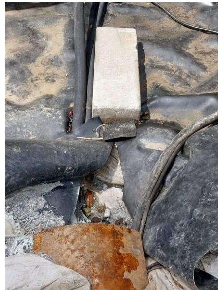
Condition of bund wall at Fuel Tank area need to be repaired
