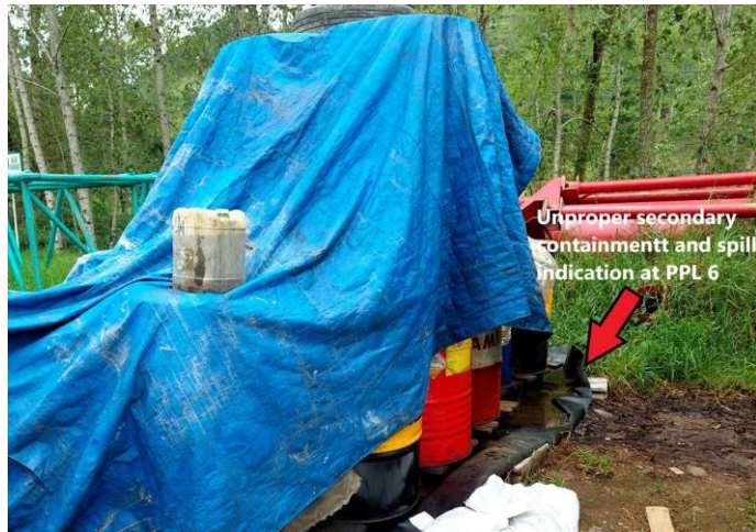
Improper B3 storage
